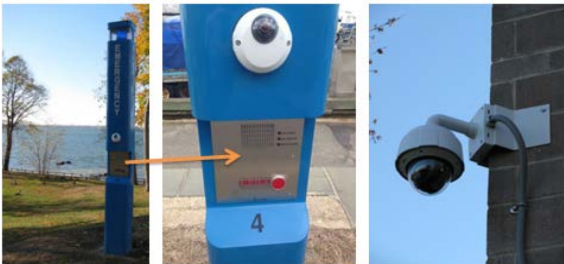
Figure 1. Call Box, Emergency Panel and Camera, and Rotational High-Definition Camera
